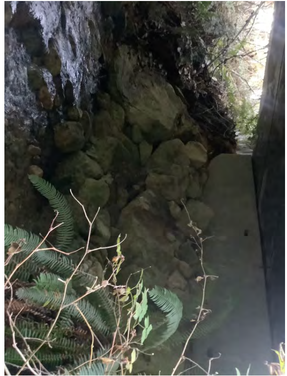
Left Bank Abutment when facing downstream
